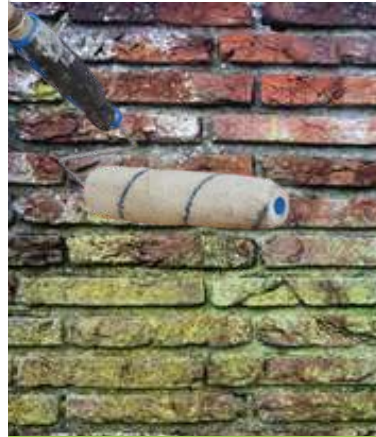
Biocidal wash applied to remove algae
