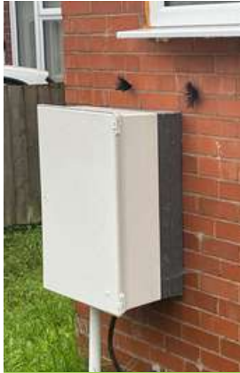
Insulation installed behind gas box which has been moved
