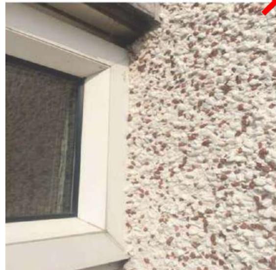
Window rendered in preventing it from opening
