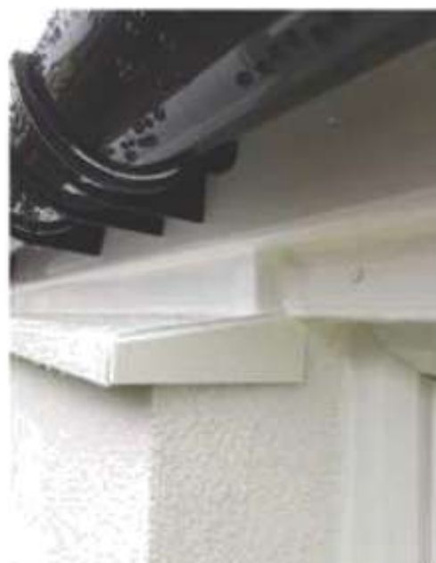
Flashings providing adequate overhang
