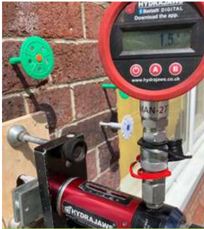
Pull out test completed to confirm fixing suitability
