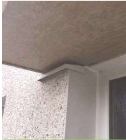
Canopy detail using a flashings and stop bead to protect the system
