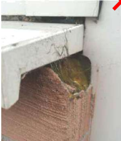
System not protected or sealed
