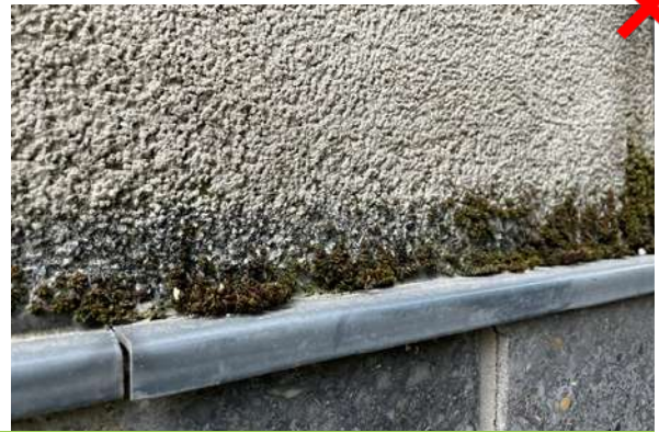
EWI Systems rendered directly down onto a flashing
