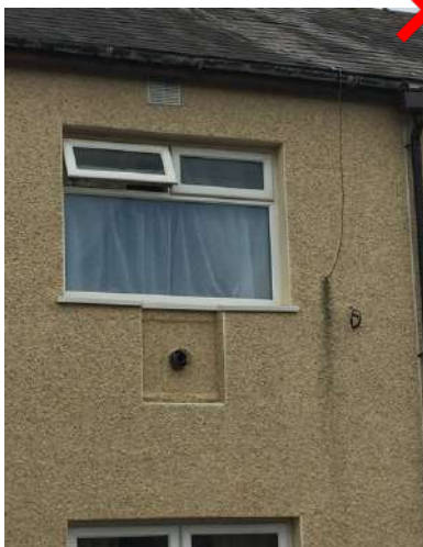
Flue under window
