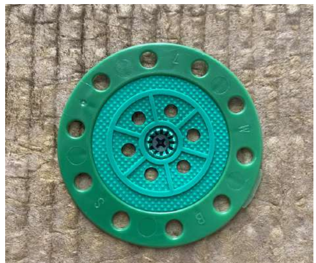
90mm insulation Washer required with Stone wool insulation
