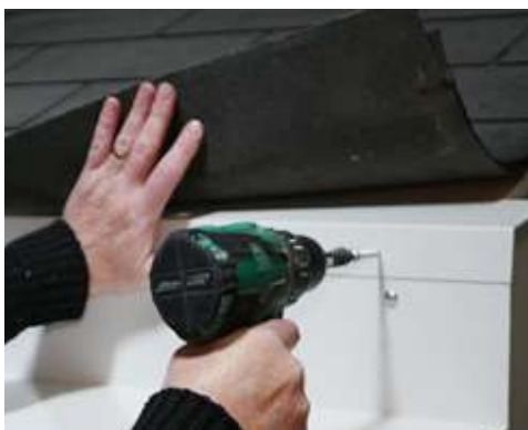
Flashing taken under existing roofing felt (where required)
