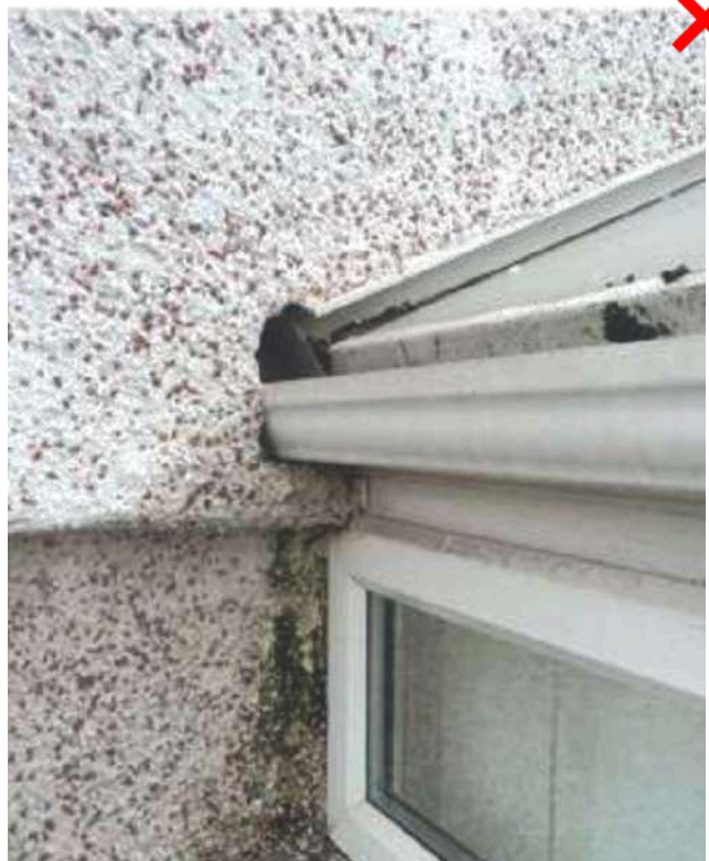
Canopies and conservatories rendered into the system creating areas for water ingress.
