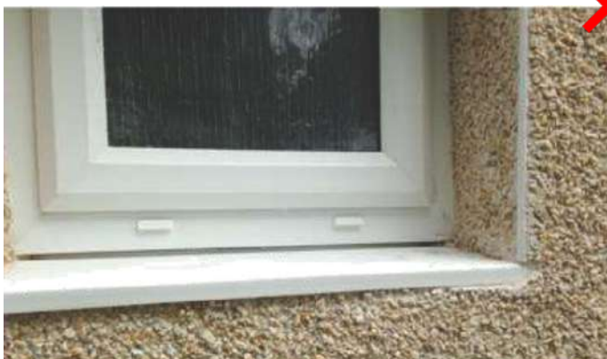
Cill rendered into system and providing no overhang/ protection.
