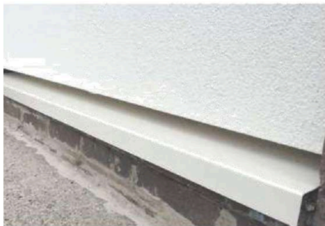
Starter track installed above a flashing
