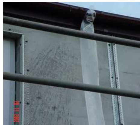
RWG sleeve used to protect EWI during installation
