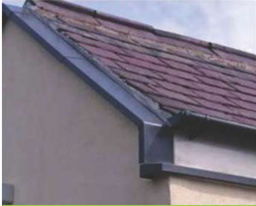
Flashings and cills providing full protection and overhang
