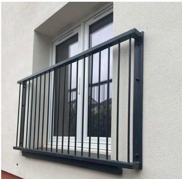
Balcony railing fixed with specialist Thermax EWI fixings
