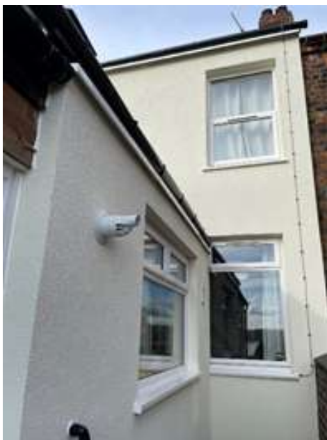
Flashings providing adequate overhang
