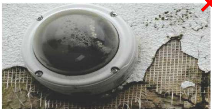
System exposed and damaged through fixing fixtures to the wall incorrectly
