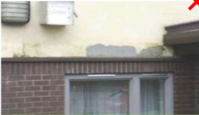
EWI Systems rendered directly down onto a flashing
