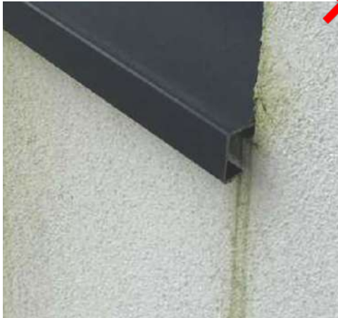
Cill too short causing staining and water ingress
