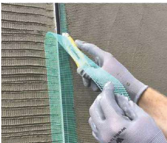
Mesh fully lapped into movement joint
