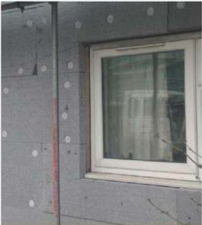
'L' shape around openings
