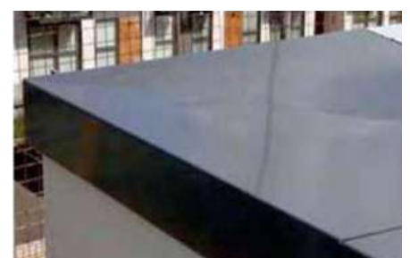
Parapet flashing
