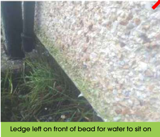
Render taken all the way to ground, starting to fail and suffering discolouration
