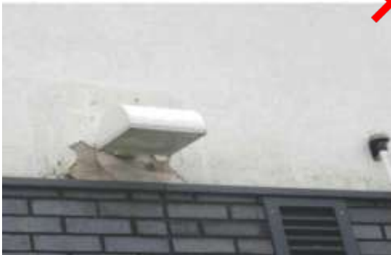
System exposed and damaged through fixing fixtures to the wall incorrectly
