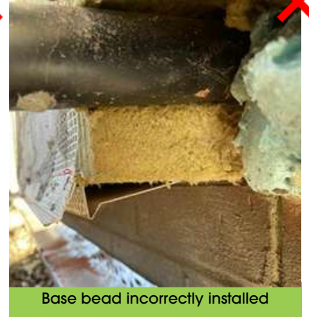
Render taken all the way to ground, starting to fail and suffering discolouration
