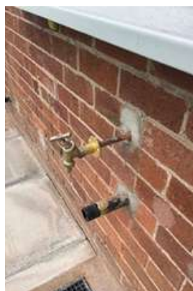
Pipework repositioned to allow for EWI system
