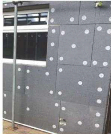
'L' shape around openings
