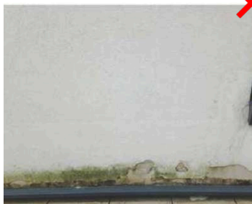
EWI Systems rendered directly down onto a flashing
