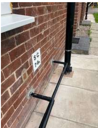
Pipework repositioned to allow for EWI system
