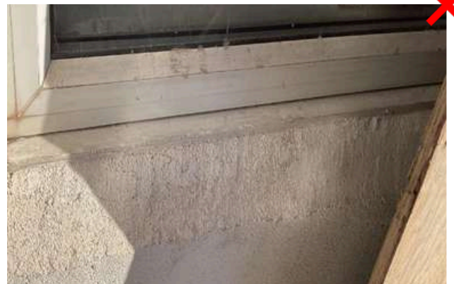
Rendered cill providing no protection
