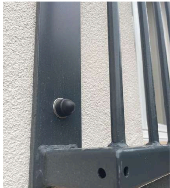
Balcony railing fixed with specialist Thermax EWI fixings
